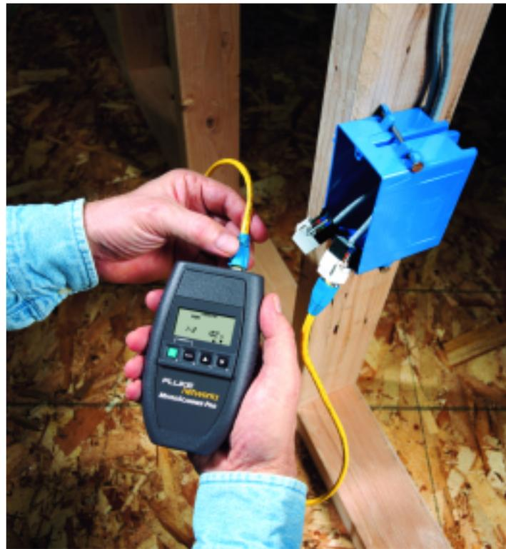
In the past, home wiring was daisy chained, meaning a cable from a distribution box was pulled from one outlet to the next until the furthest outlet was reached and terminated. However, if one connection fails then all those beyond it fail. This won't cut it anymore with the high-speed data requirements of technology savvy homeowners. Today's preferred layout relies on “home runs,” dedicated cable runs to each outlet so that each functions independently.
