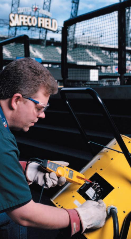
Akres and Wolford depend on Fluke test equipment to make sure the roof's moving parts stay in championship shape. Their T5-1000 electrical testers ride next to their pens in their shirt pockets, pulled out throughout the day to quickly test whether a circuit is dead or alive. A Fluke 177 digital multimeter checks voltages in the systems' many junction boxes, probing for shorts, and a Fluke 1520 helps the crew conduct its motor insulation tests.
