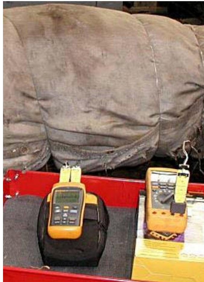
After a welding repair, it is essential to perform a stress relief to maintain the integrity of the steel.
