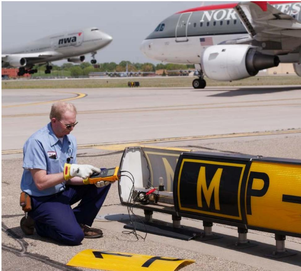
MSP electrical foreman, Mark Temple, uses a Fluke 1520 MegOhmMeter to locate trouble spots.
