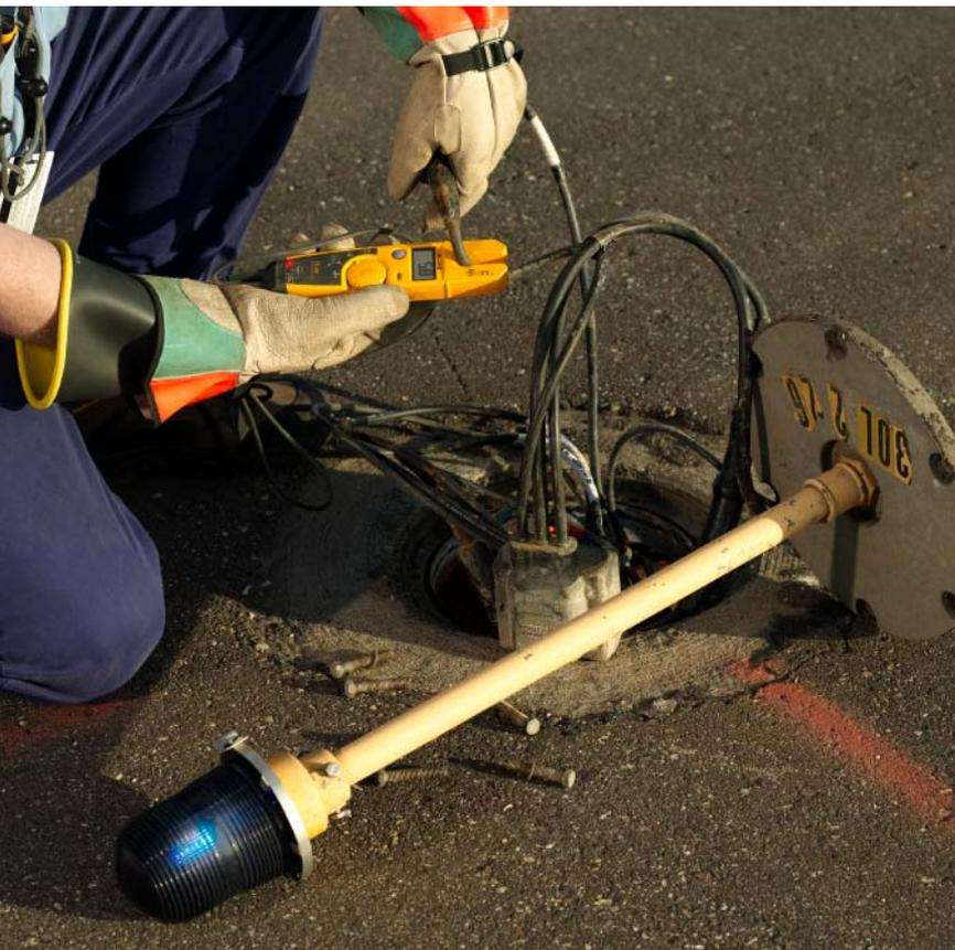
Using a Fluke T5-1000 electrical tester to check current.
