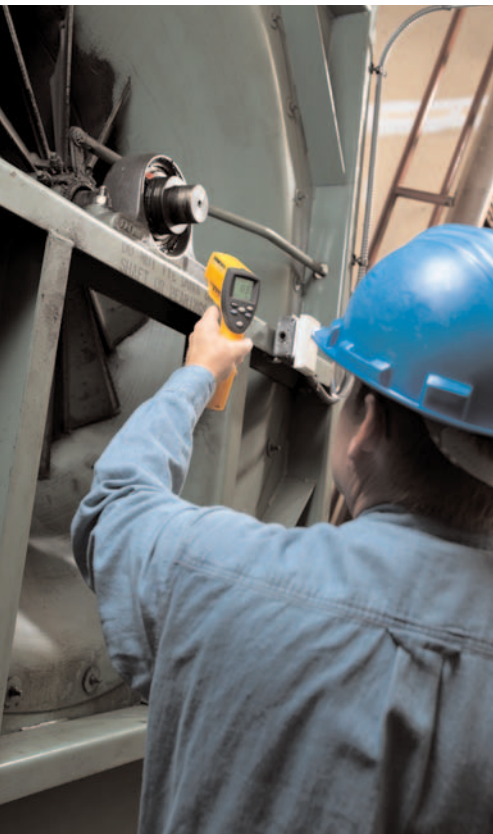
Using an infrared thermometer to quickly measure bearing heat.
