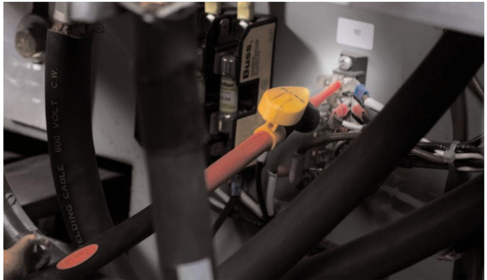
When working in a deep or recessed panel, use a test probe extender and probe light to illuminate the area.
