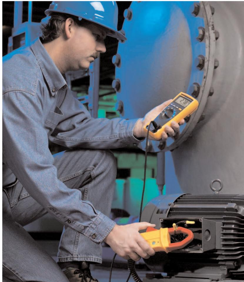
Measuring current with a Fluke-179 DMM and current clamp.
