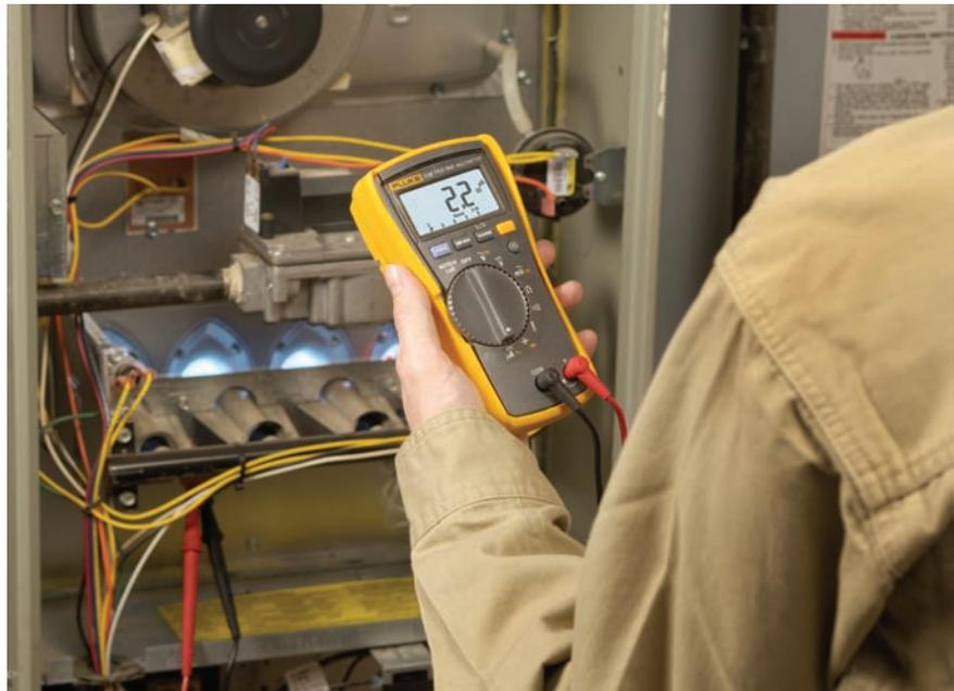
DMM with microamps capability testing the flame rectification circuit.
