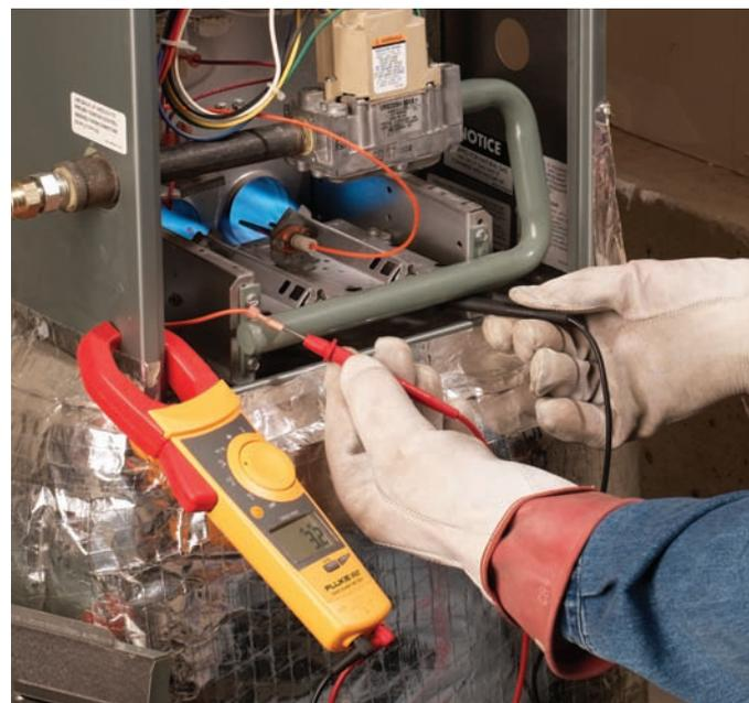
Testing voltage with a multi-function clamp meter.
