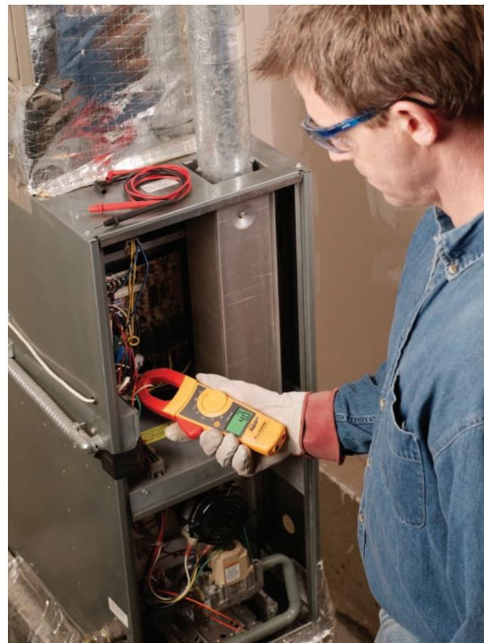
Checking current with a clamp meter.
