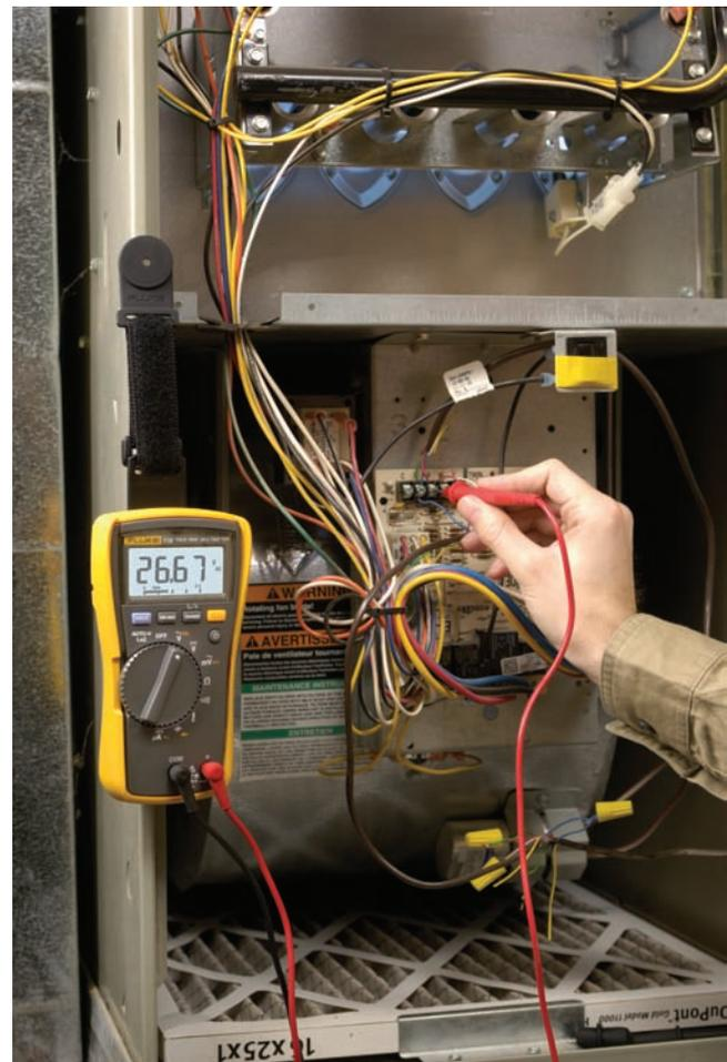
Checking the 24 V ac supply voltage.
