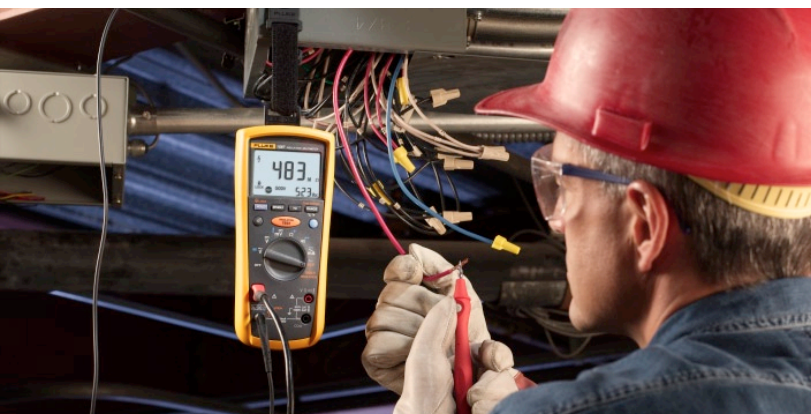
Avoid electrical shorts by testing the insulation resistance on cabling.
