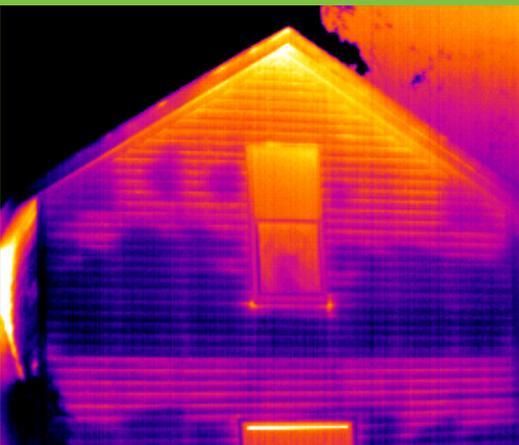
Inspecting to locate air leakage requires a 4 °F or higher temperature difference between inside and outside air, in order to get accurate readings. Air leakage can be into the building, as in the cold air shown leaking through the floor, or out of it, as in the warm air leaking out alongside the roof peak.
