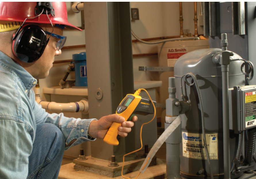
Taking a contact temperature measurement at the compressor outlet on the liquid line.
