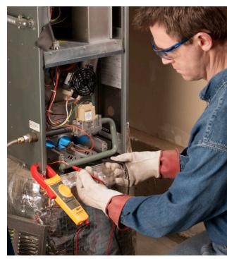
Testing the flame rectification circuit on a residential furnace.
