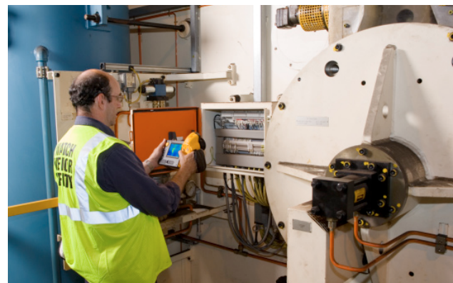
Chuck Larabell inspecting the Schuler Press Main Motor Control.
