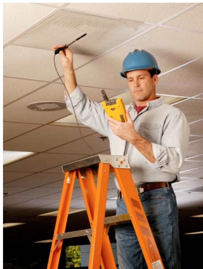
Measuring air flow at a supply register.
