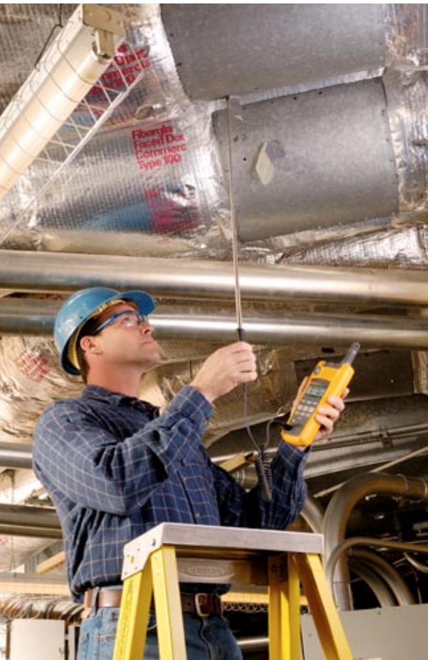
Measuring air velocity in a duct.
