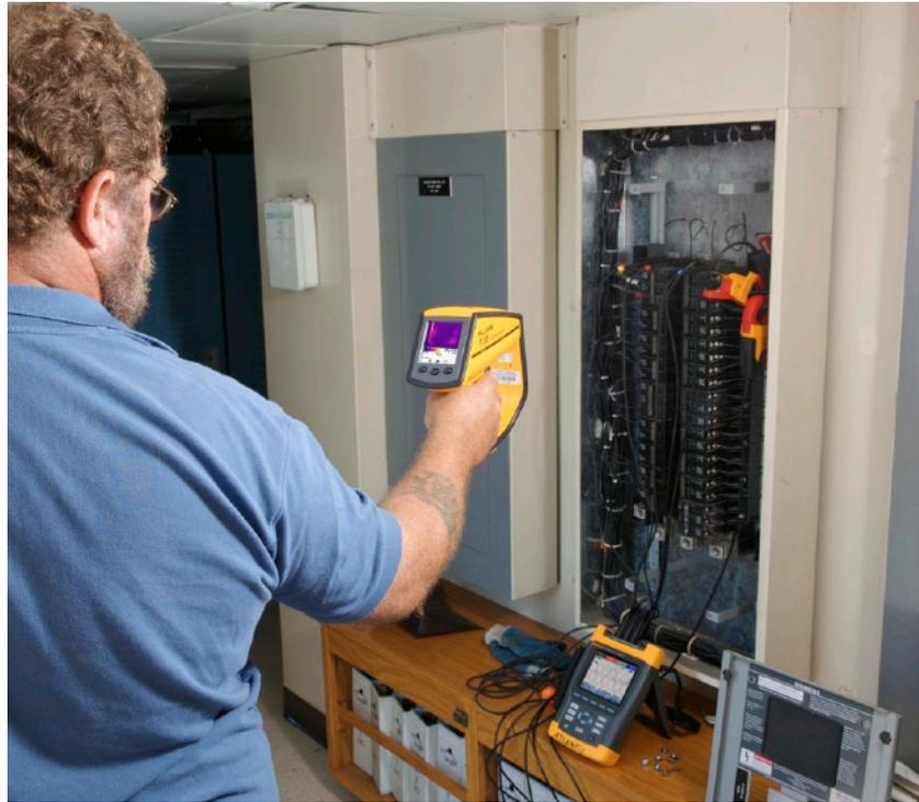
**Tools:** Fluke 434 Power Quality Analyzer, Fluke Ti30 Thermal Imager
