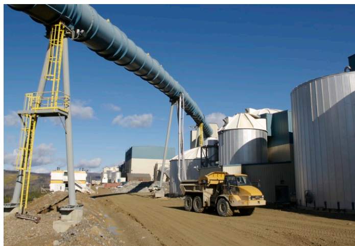
Looking north at the Mill and Filter building facilities. In the blue tube is the conveyor belt that brings the ore from underground to the mill.
