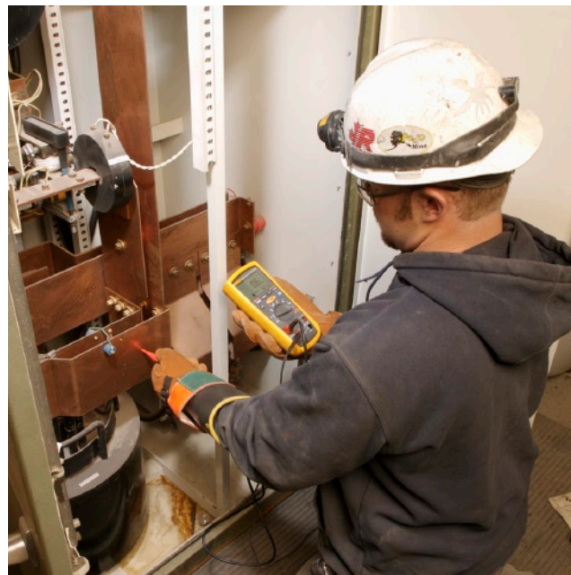
Checking incoming bus voltage and troubleshooting one of the mill's primary breakers.
