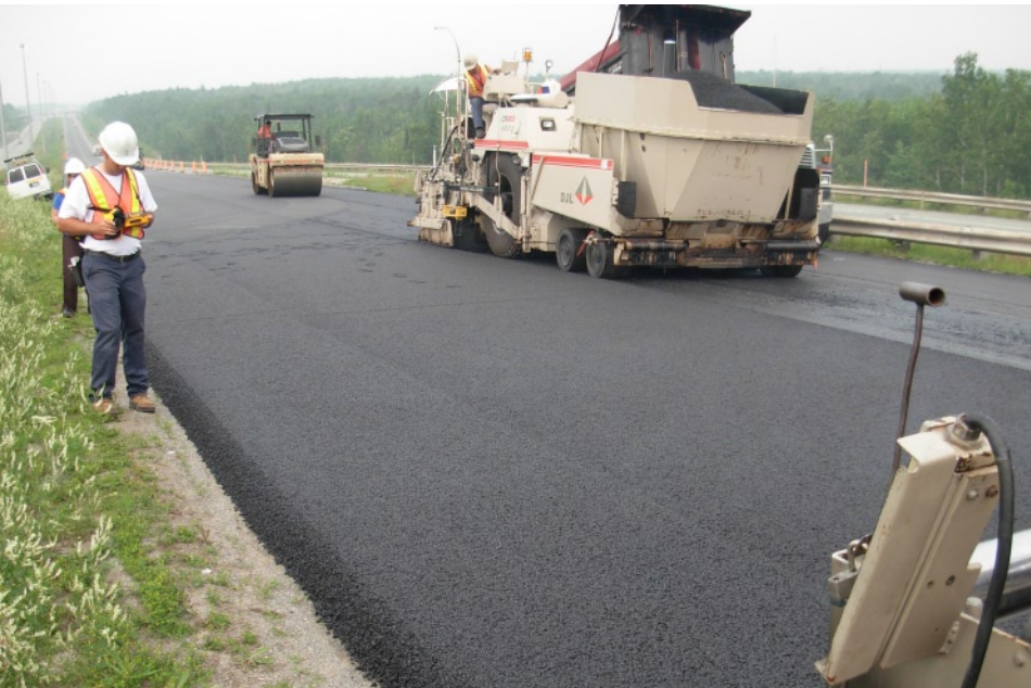
Taking asphalt temperatures during application.
