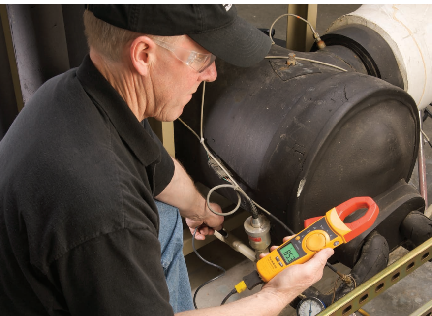
Liquid line temperature measurements for subcooling.
