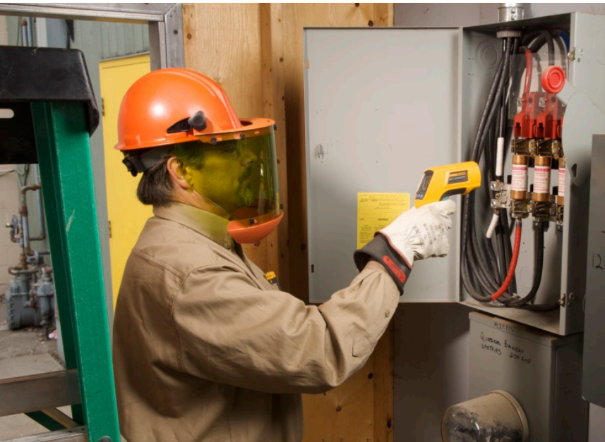
Jim Turner comparing infrared heat signatures across three phases.
