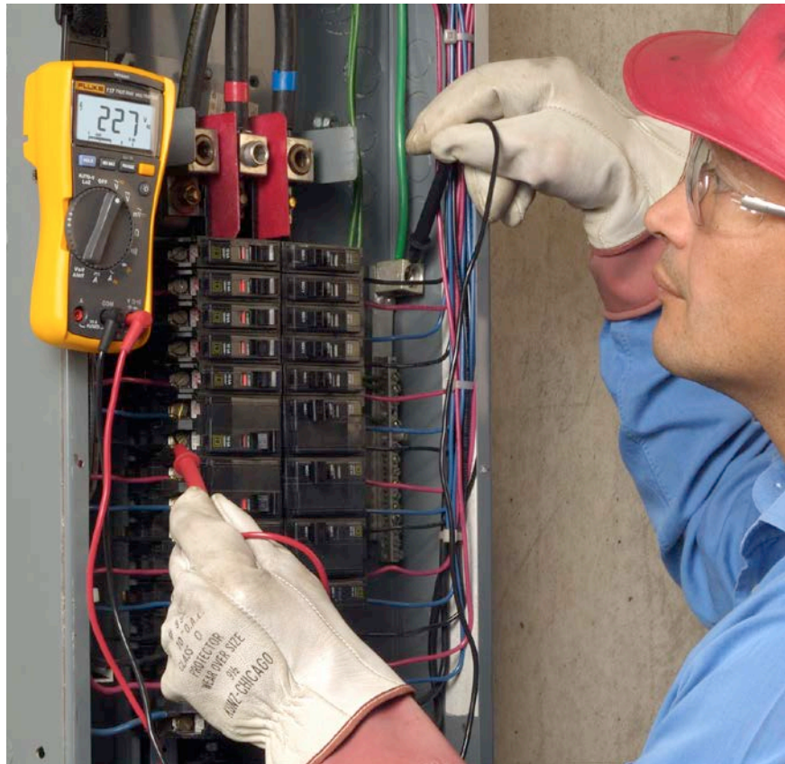
Figure 3. A DMM with a low-impedance option is the smartest pick for a live-dead-live test.
