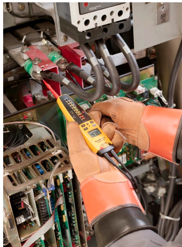
Depending on the application, technicians use the LED voltage light indicators, the vibration feature, or the LCD voltage readout.
