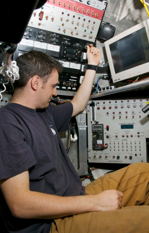
Sean Kelley switches through the various electrical systems aboard the sub, and compares the analog meters against the Fluke 77 DMM mounted in the control panel.
