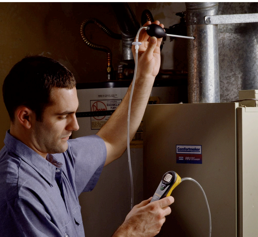
Taking Flue gas samples with the CO-220 Carbon Monoxide Meter and CO-205 Aspirator Kit.
