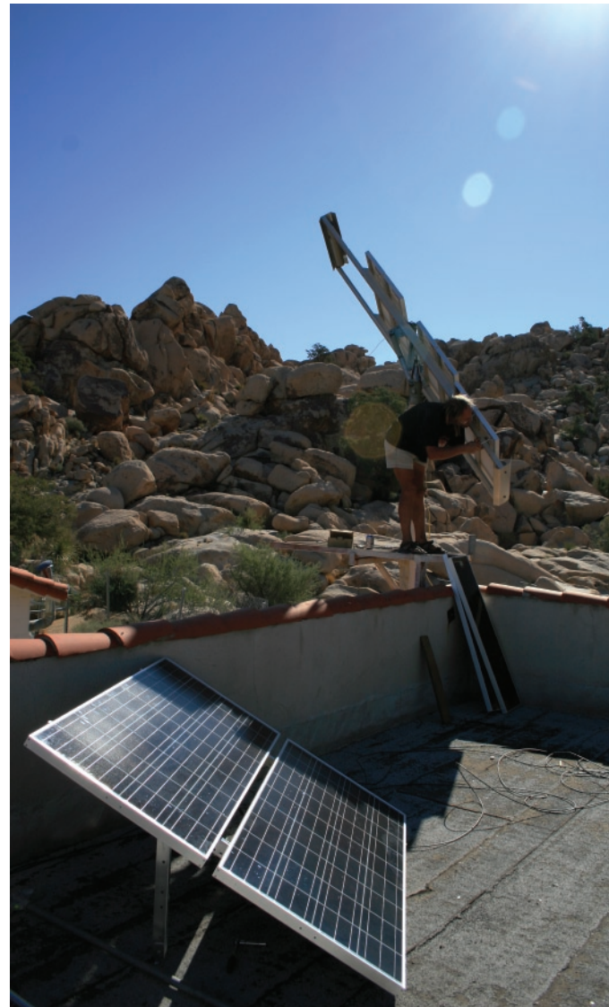
Testing a solar installation in Joshua Tree.
