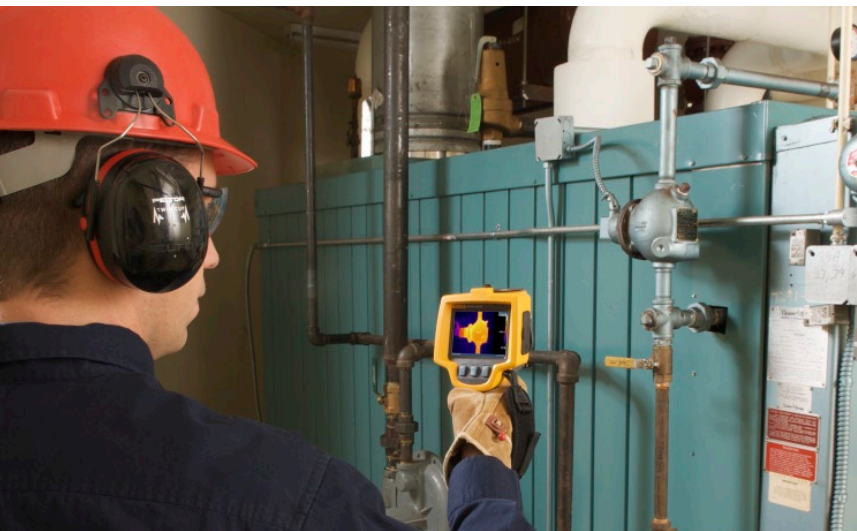
If your facility uses a boiler, scan the steam lines to check for leaks, blockages, and failed traps.
