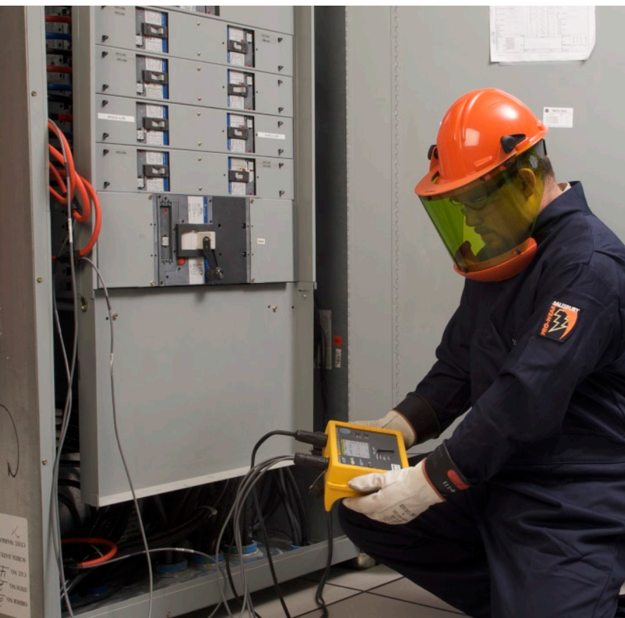
Testing power on a distribution panel.
