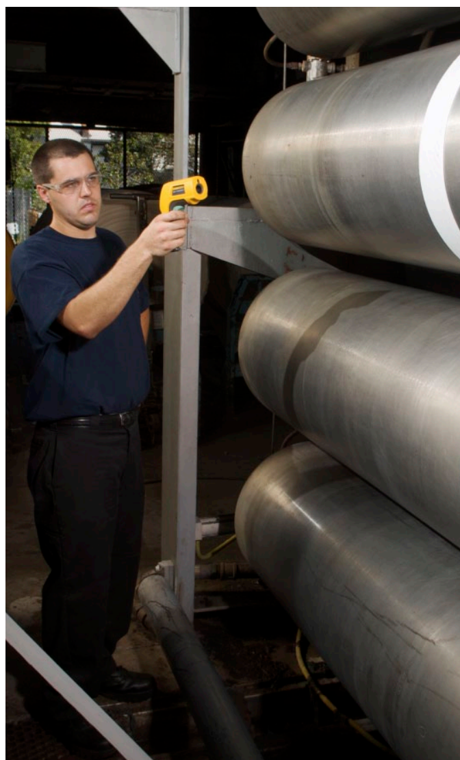
Tom uses the Fluke 568 to look at the temperature of the drying drums in between fabric runs. The operator can dial in the temperature on the cans by setting the steam pressure. The typical temperature range is 215 °F to 275 °F.
