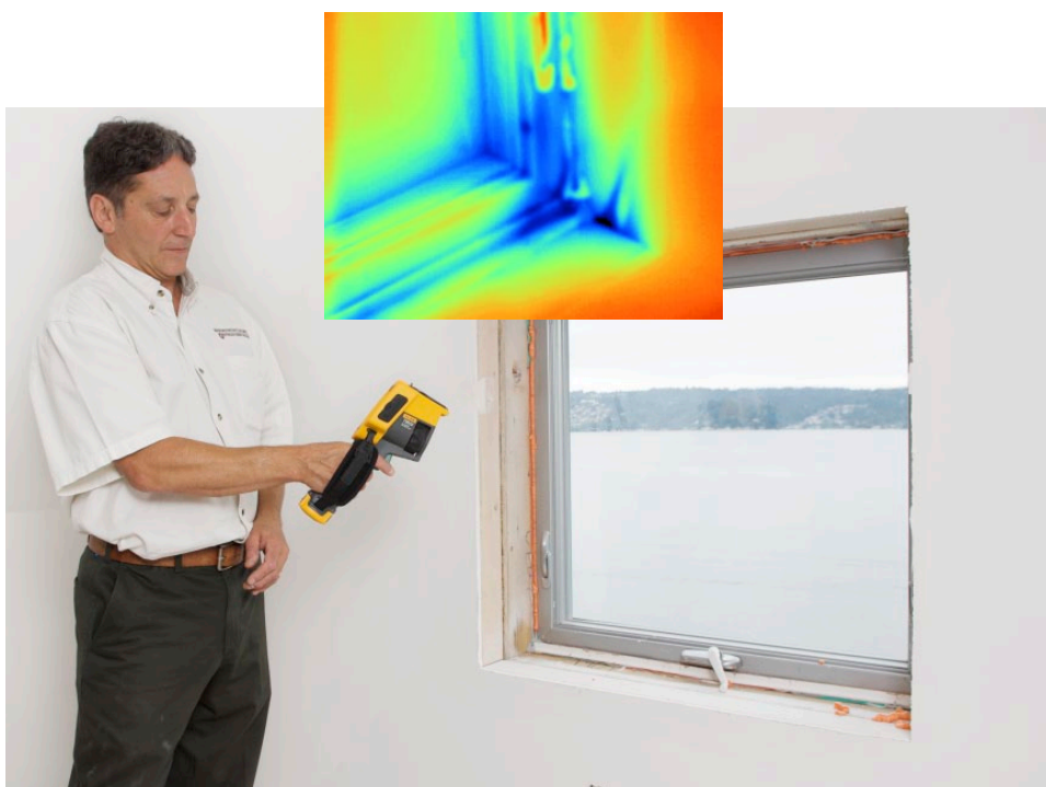
Inspecting all windows, doors and envelope penetrations from the inside of the house also yielded interesting information that helped to further increase the home’s energy efficiency.
