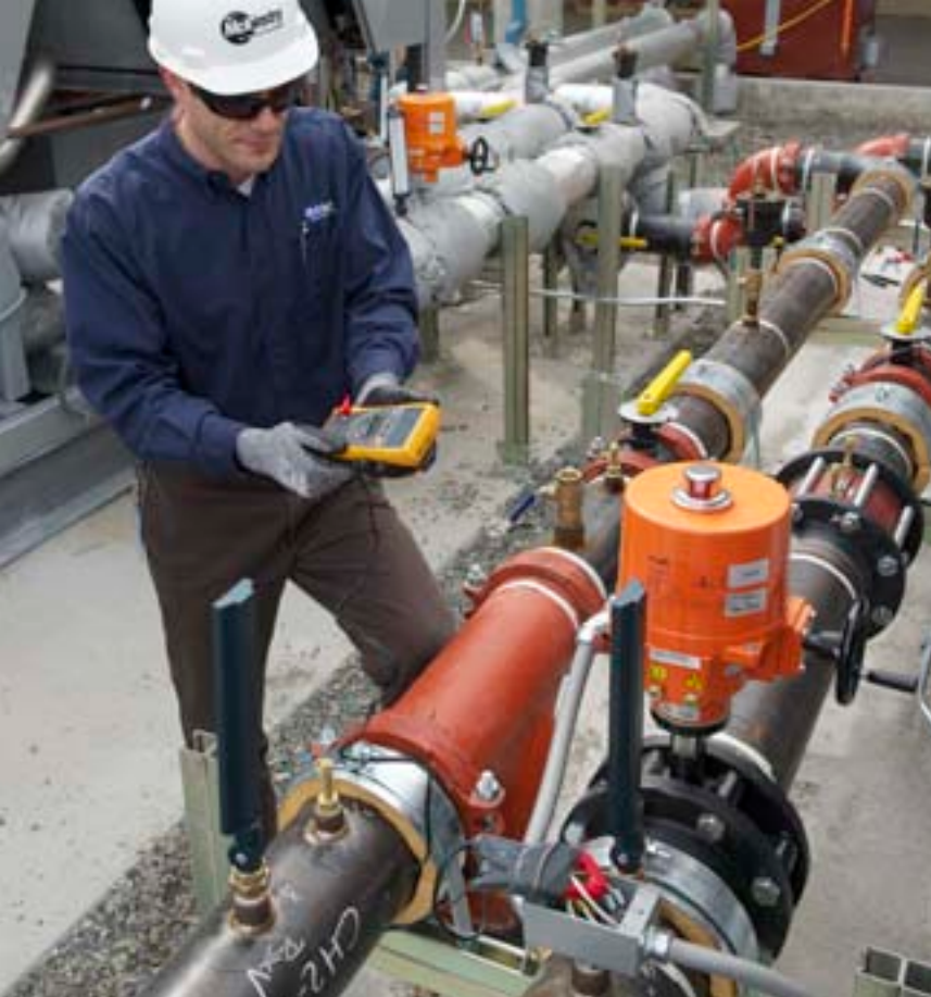
Commissioning engineer Jeff Fogel uses a multimeter and clamp accessory to verify chilled water valve operation.
