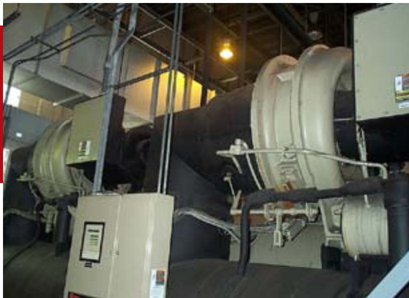
Commonly, a group of centrifugal chillers provides redundancy and step capacity.
