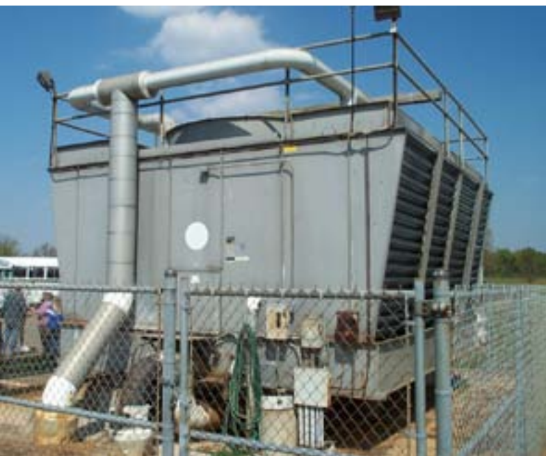
The insulation and windings on cooling tower fan motors must be tested.
