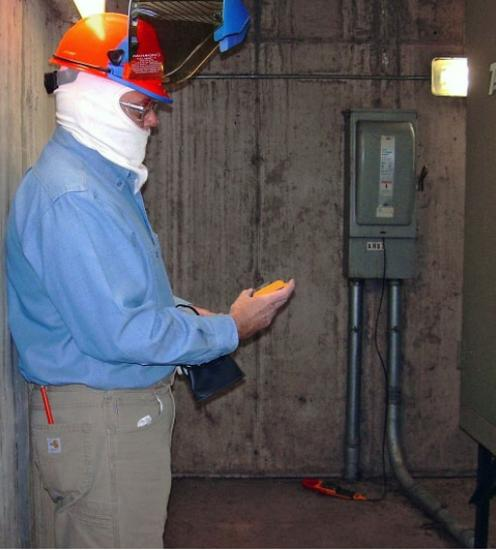
**Figure 3.** The Fluke iFlex™ probe has been placed around the incoming 480 V conductor and the disconnect door closed, though not latched. The Fluke 381 clamp meter lies on the floor beneath the disconnect. With the remote display unit removed from the meter, the instructor is able to remain well outside of protective boundaries to observe, demonstrate, and discuss readings.
