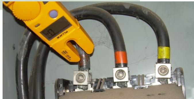
**Figure 1.** Selecting the proper test equipment for the job is a basic requirement for electrical maintenance, and is identified as such in NFPA 70B. Here we quickly determine that the Fluke T5 is too small for the 250 kcmil conductors. On-the-job training, as well as actual maintenance, requires a meter that will provide accurate readings and enhance safety.
