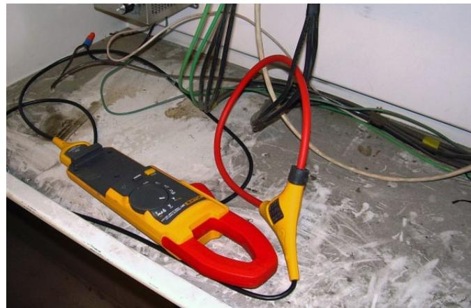
**Figure 2.** One advantage of the iFlex™ probe is its ability to pass through and around conductors with little disturbance to the conductors. Here the Fluke 381 is lying in the bottom of the AHU VFD cabinet and is connected to read current to the drive. The remote display unit has been removed to allow readings to be taken with the enclosure door closed.
