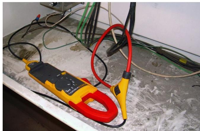
**Figure 2.** One advantage of the iFlex™ probe is its ability to pass through and around conductors with little disturbance to the conductors. Here the Fluke 381 is lying in the bottom of the AHU VFD cabinet and is connected to read current to the drive. The remote display unit has been removed to allow readings to be taken with the enclosure door closed.
