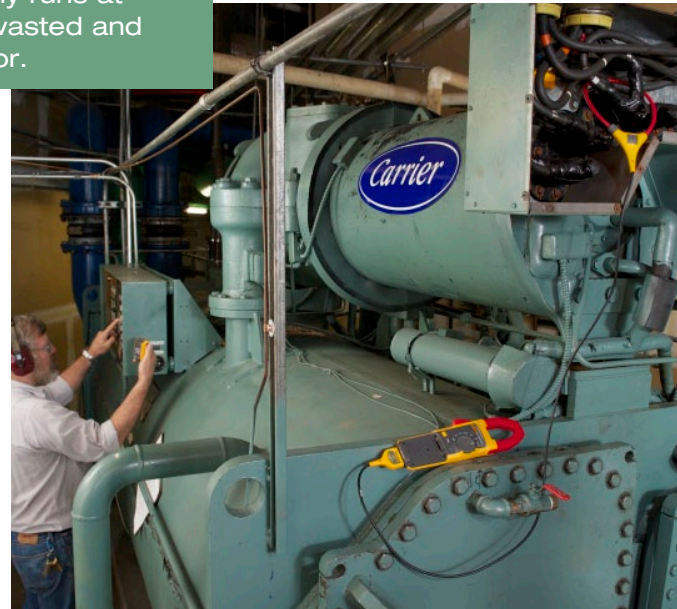
Run a Fluke iFlex™ Fluke Current Probe around a single conductor. Or, you can center the jaws of a clamp meter around a single conductor.
