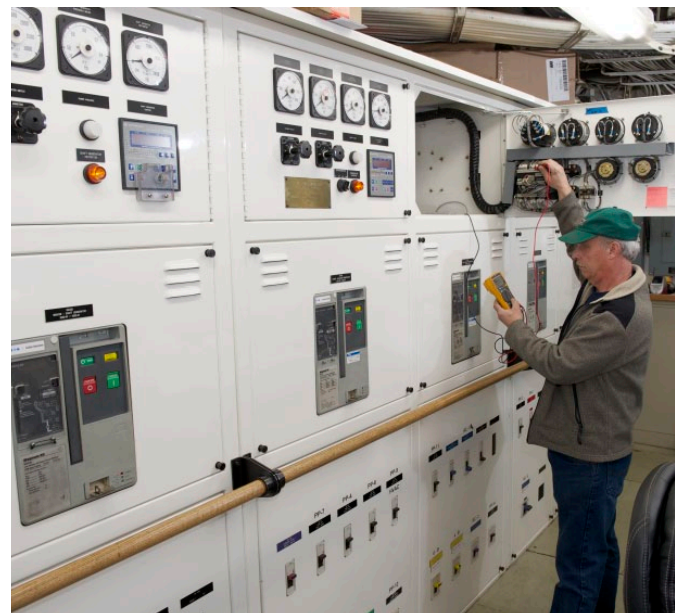
Jim Potts tests continuity in the power control panels Harris built and installed deep in the Starbound's interior.
