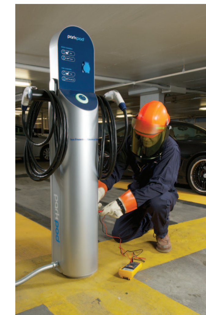
Keith Wood checks the voltage available at the ParkPod charging station, using his Fluke 1587 Insulation Multimeter.
