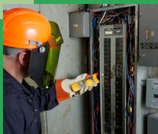
Wood uses his Fluke 337 Clamp Meter to verify that amperage available at the panel is adequate to supply the charging station.
