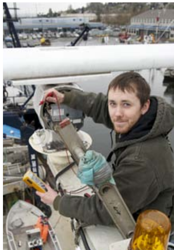
High above the harbor, field electronics technician Jeff McMahon tests power supplied to a radar antenna.
