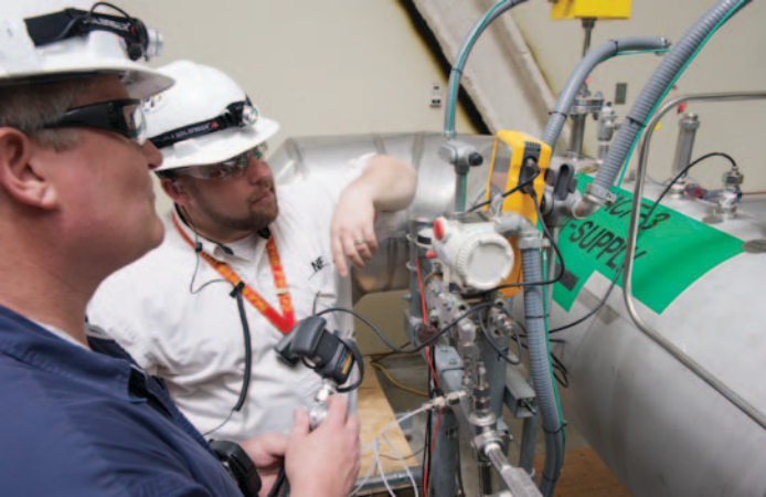
Travis Averill and Mark Jensen at a test point. To maintain precision performance, every test point is on a schedule to be tested and calibrated.
