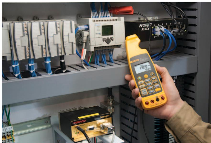
Figure 4. Measuring current on a 4-20 milliamp process control loop.
