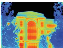
Energy losses are common in commercial buildings and industrial facilities. While there can be a number of culprits, such as air leaks or systems running inefficiently, many energy losses can be detected through inspection with thermal imaging.
