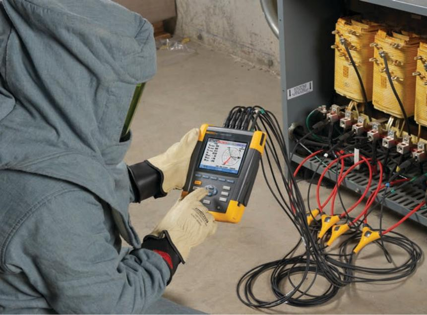
Use a power quality analyzer, such as this Fluke 435 Series II Power Quality and Energy Analyzer, to measure and record the specific parameters associated with power quality.
