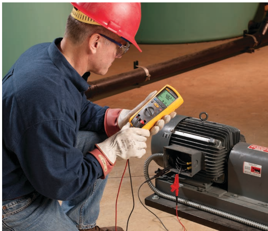
Taking insulation resistance tests.
