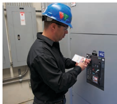
Zach Bryson, Project Manager for Keithly Electric, locks out and tags the power supply at iFLY Seattle. Initial inspection will proceed with the facility de-energized.
