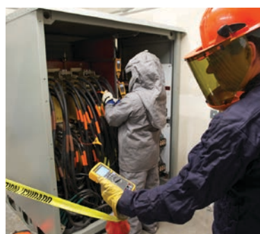
Working outside the limited approach boundary, Burdick (foreground) reviews readings on the Fluke CNX wireless system as Bryson works in the background.
