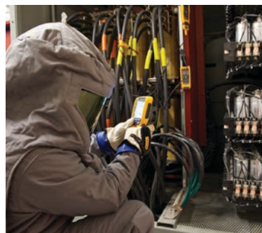
Bryson uses a Fluke CNX compatible infrared camera to inspect fuses and power capacitors while the system is under load.
