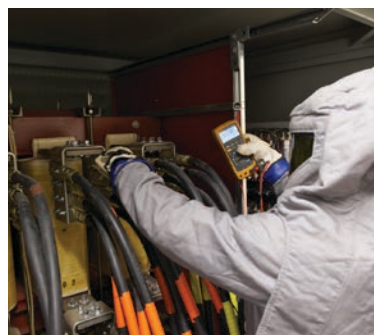
Suited up for arc flash safety, Bryson uses two separate Fluke 87V Industrial Multimeters to verify that all sources of energy were isolated by lockout. The team used two meters—checking phase-to-phase and phase-to-ground with each meter to verify all sources of energy have been discharged (capacitor bank).
