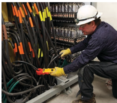
After verifying that all sources of energy have been isolated, Keithly technician Greg Burdick uses the Fluke 1630 Earth Ground Clamp Meter to check grounding at the harmonics filter.
