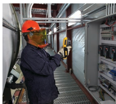
Burdick uses a Fluke infrared camera to inspect the variable frequency drive control panel for the iFLY louver system.
