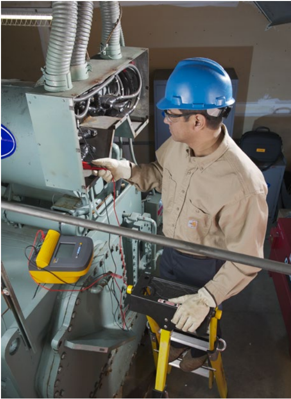
Insulation resistance testing with the Fluke 1555
