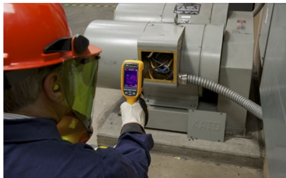
Performing an infrared inspection with the Fluke Ti125 Industrial-Commercial Thermal Imager
