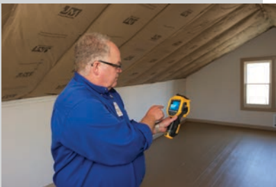
Quickly inspect for any insulation gaps or damage.
