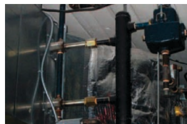
This image shows the steam feed, into the HVAC duct. The feed tube shows condensation in the bottom of the vertical tube.
