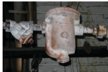
When operating correctly as here, steam trap thermal images should show an abrupt change in temperature.
