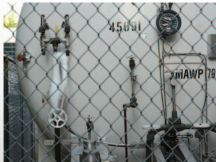
Difficult inspection sites
