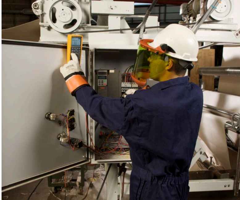
Wearing appropriate PPE, test a known live source to verify meter functionality and then test the panel for absence of voltage, all before declaring it de-energized.
