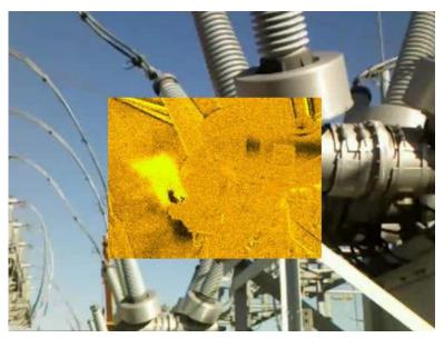
Figure 2: A thermal image with gas detection overlaid on a visible light image of a circuit breaker.
