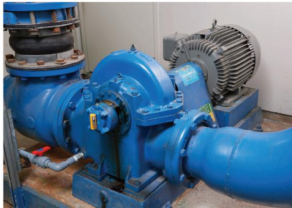
If a pump's impeller is imbalanced, vibration will occur, and the pump's performance and efficiency will be adversely affected, with poor production and excess costs. With time, the imbalance will cause pump failure. If the baseplate or foundation is uneven or if one of the motor's feet is uneven, soft foot can occur, causing excess vibration. In worst-case scenarios, imbalance left unchecked can lead to cracked or broken shafts, which can be personnel safety hazards.
