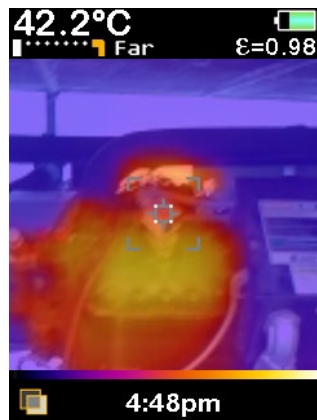
One of the Operational Stages
